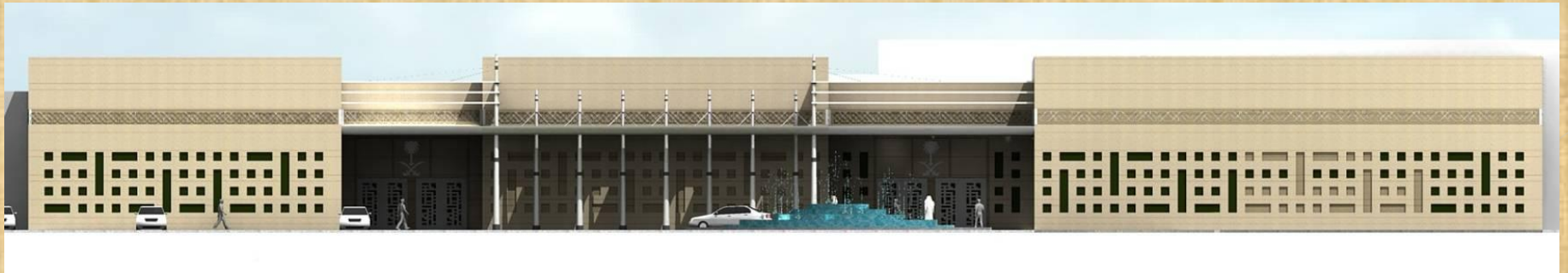
Building Main Facade
